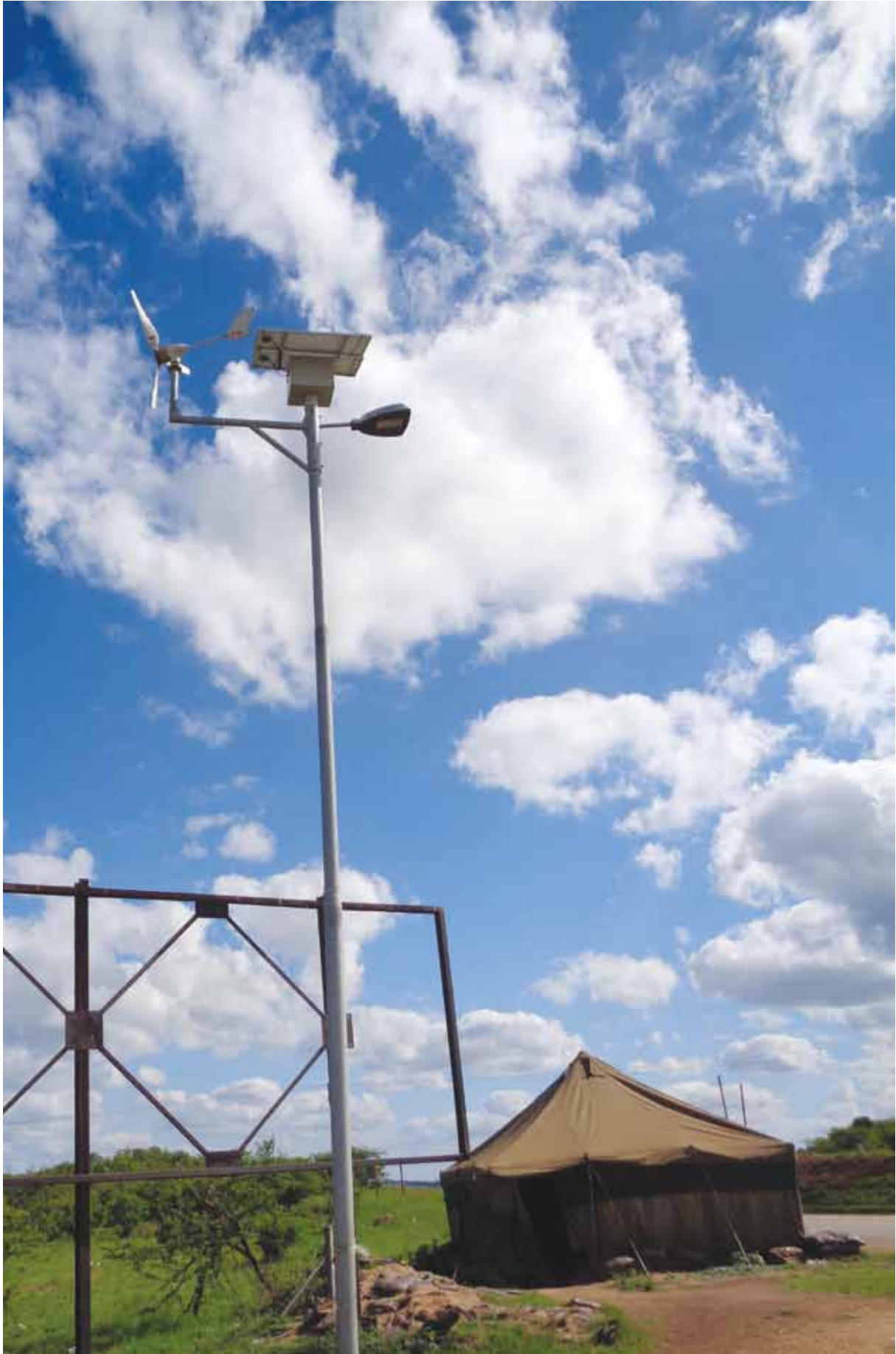
Wind and solar hybrid security light at a military checkpoint along the road between Siteki and Mhkumeni
