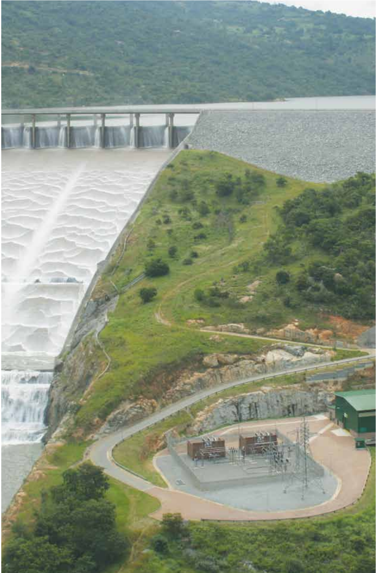
The Maguga 20MW Hydropower Station
