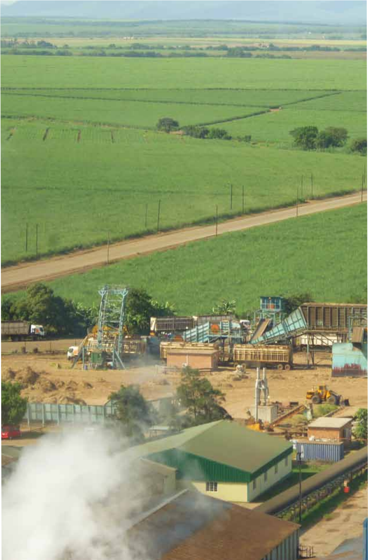
Ubombo sugar cogeneration plant
