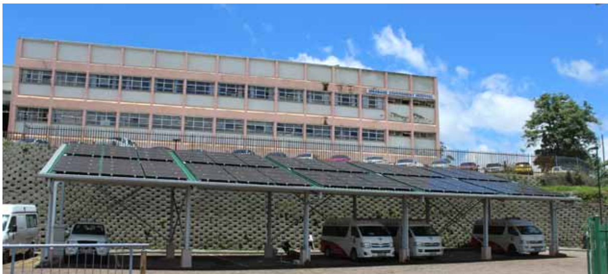
A 32 kW solar PV powering the blood bank in the Mbabane Government Hospital
