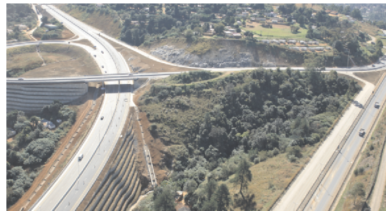
Aerial View of the Mbabane Bypass Road (MR3)
