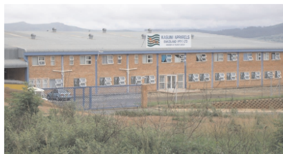
Government factory shell at Matsapha rented to Kasumi Apparels Swaziland (Pty) Ltd
