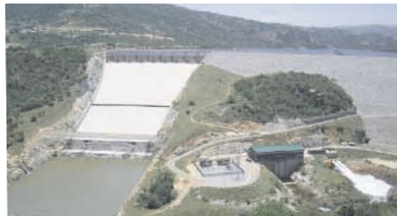
Maguga Power Station
